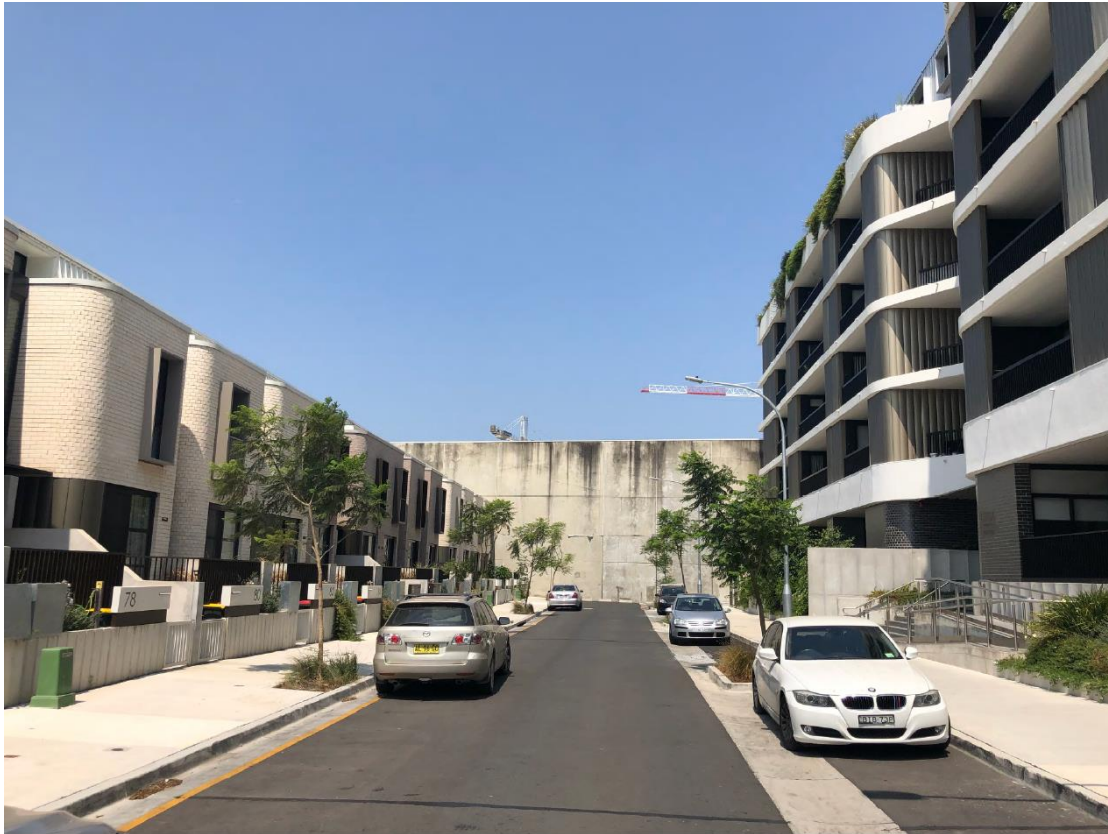
Figure 5: The existing warehouse in the distance from Metters Street looking east
